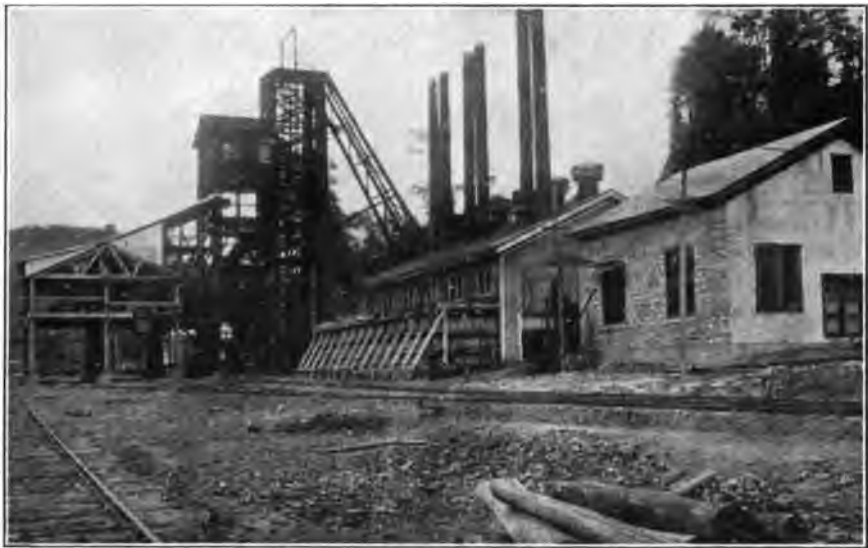
PLATE XXVIII(b).—Mines Nos. 1 and 2 of New River Collieries Co. at Eccles.
